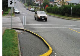
Temporary rubber curb extension in British Columbia
