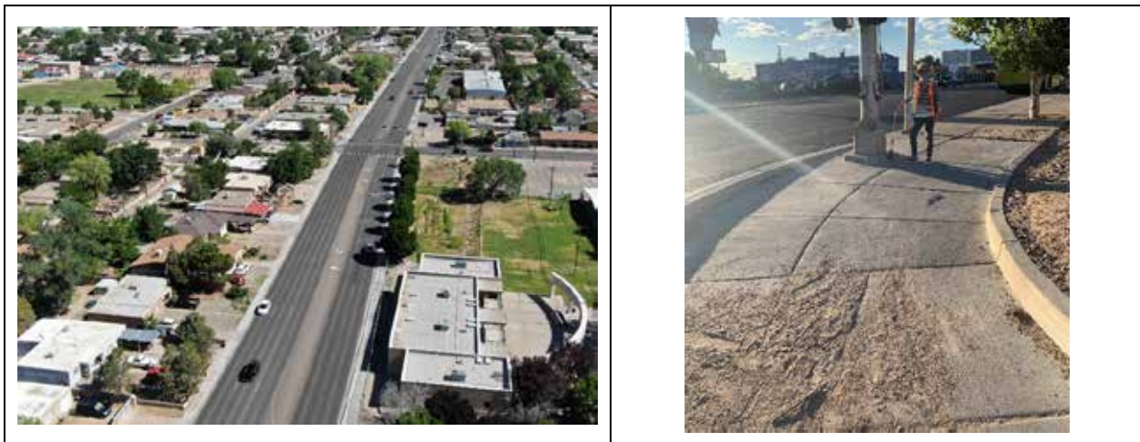
Left Image: A photo, looking north, showing the five travel lane and TWLTL median cross section. Credit – City of Albuquerque. Right Image: A photo of one of the corridor's signalized intersections with sand and stone debris in the curb ramp area. Credit – City of Albuquerque.
