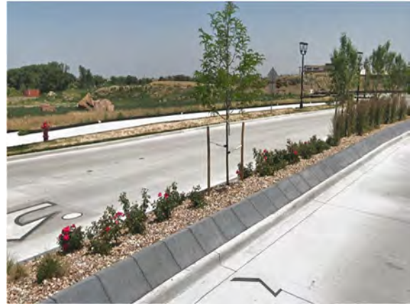
Median Treatment to Discourage Pedestrian Use
