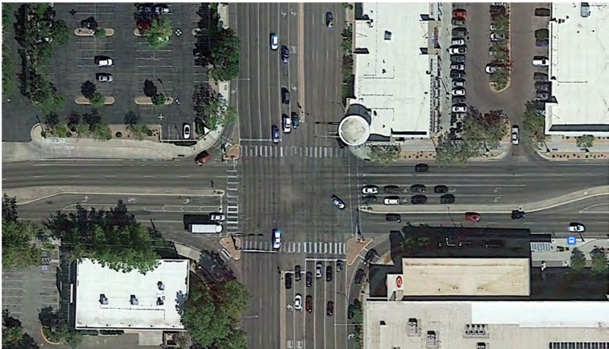
Figure 2-1. Existing Roadway at Louisiana
