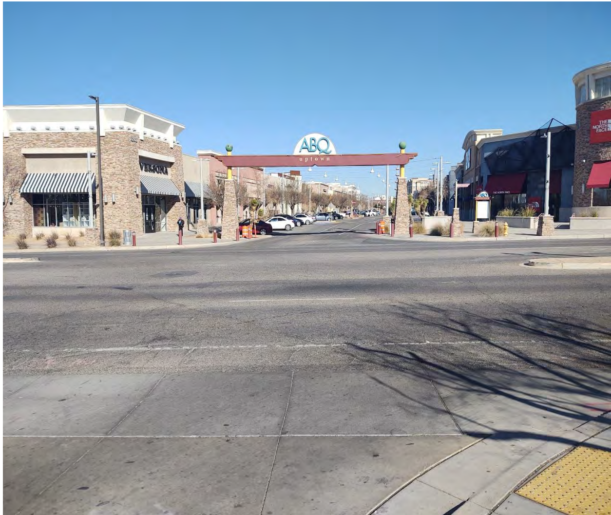
Photo 3: Indian School Road at Q Street - Looking North. Low severity raveling, oxidation, and weathering. Low severity to moderate transverse cracking of asphalt concrete.
