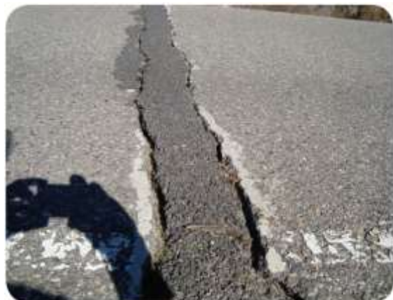
Figure 74: Pavement Crack Repair Using Rigid Material, Pulling Away from
