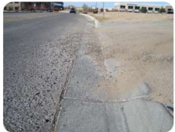
Figure 71: Unwanted Gravel and Sand on a Bike Route from Unpaved Driveway
