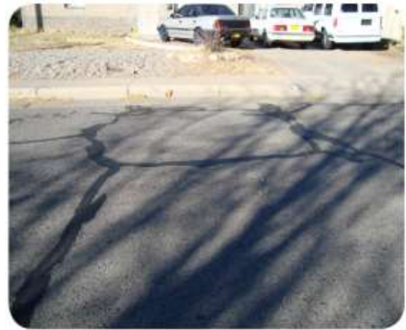
Figure 68: Crack Sealed Pavement
