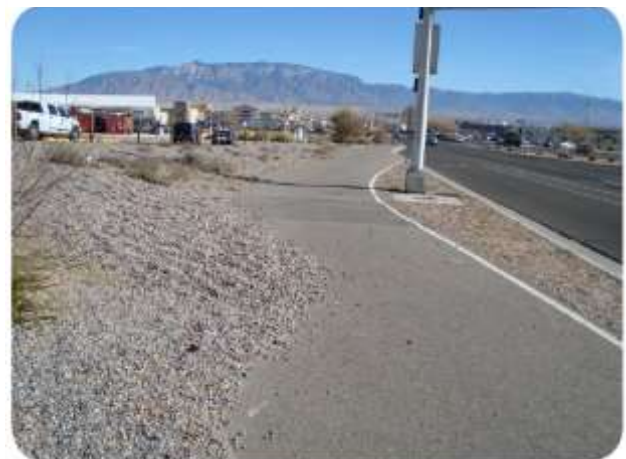
Figure 78: Landscape Gravel on Adjacent Side Slope Migrating onto Trail
