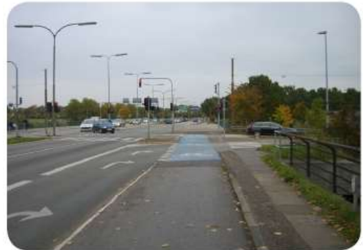
At this unsignalled right turn, the cycle track has dropped to a bike lane with blue coloration and pavement markings through the conflict area.
