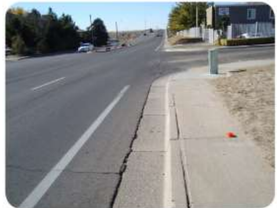
Figure 71: Unwanted Gravel and Sand on a Bike Route from Unpaved Driveway
