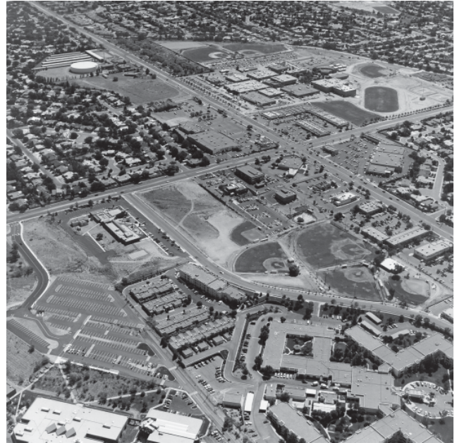
Figure 13: Typical major arterial intersection and auto-oriented land use.
