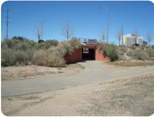
Figure 15: Concrete Box Underpass Structure beneath an Urban Principal Arterial
