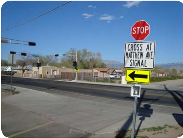
Figure 18: Multi-use Trail Diverted to Signalized Intersection Crossing.
