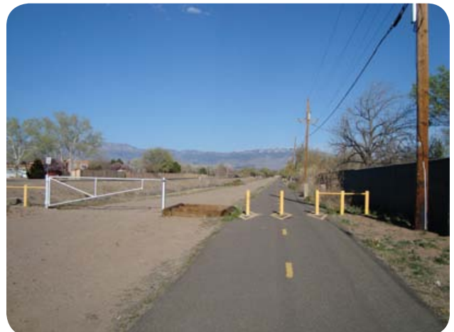
Figure 29 Multi-use Trail Sharing a Utility Easement Along the Alameda Drain in the Near North Valley.
