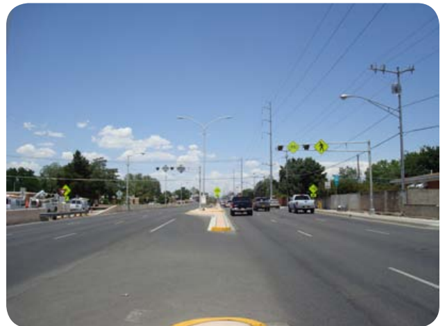
Figure 21: Multi-use Trail Mid-block Crossing of Wyoming Blvd. a Six-lane Principal Arterial.
