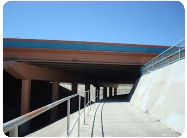
Figure 16: A Notch along the Drainage Channel Providing Multi-use Trail Access Under I-40
