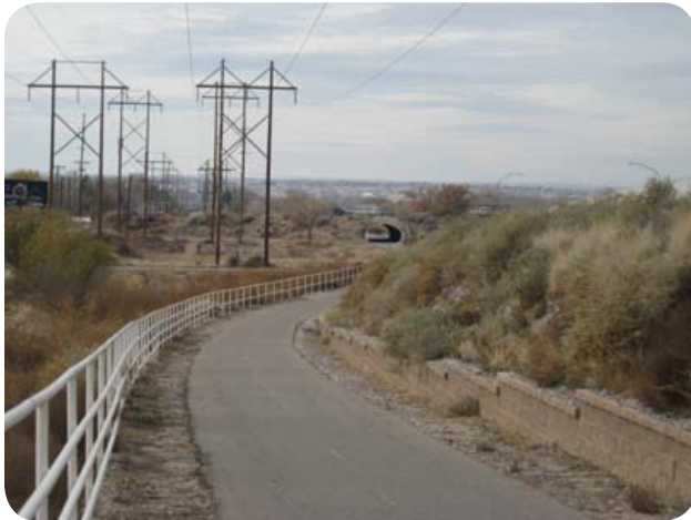
Figure 17: Multi-use Trail with Corrugated Multi-plate Type Underpass crossing 4th St.
