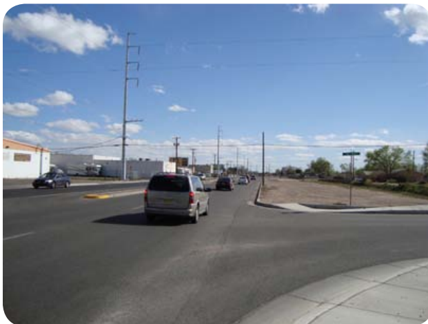
Figure 4: Wide shared outside lane
