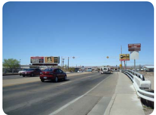
Figure 3: Typical bike lane on roadway bridge
