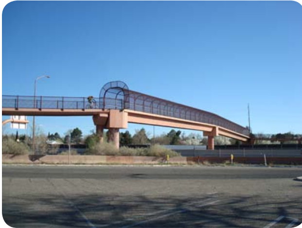
Figure 11: I-40 Overpass Near Uptown
