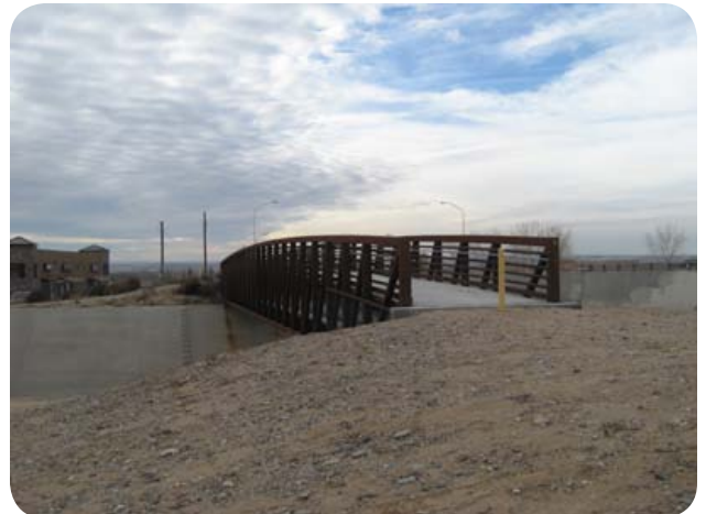
Figure 14: Single Span Pre-fabricated Truss Bridge Crossing Drainage Channel
