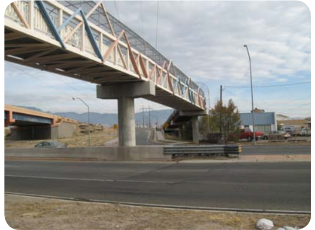
Figure 12: Paseo del Norte Multi-use Trail Overpass crossing 2nd Street
