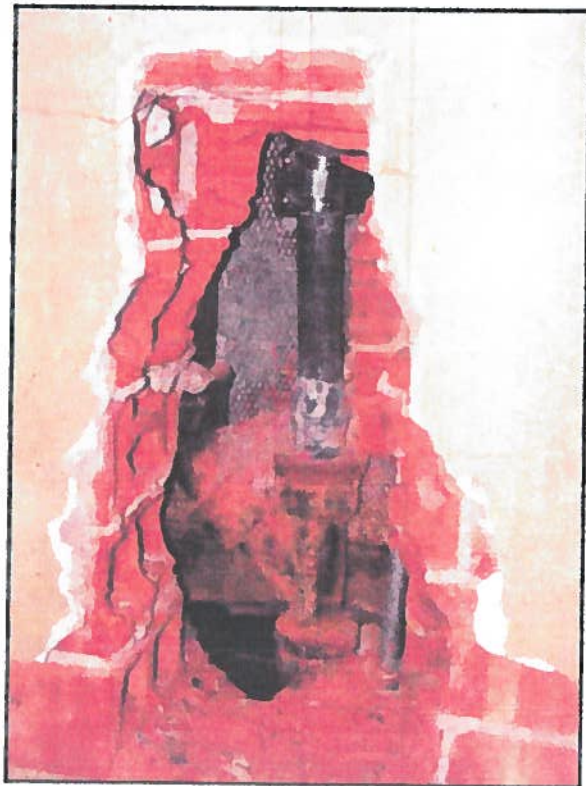
Fig. 20. Opening in exterior wall and bathroom pipes.
