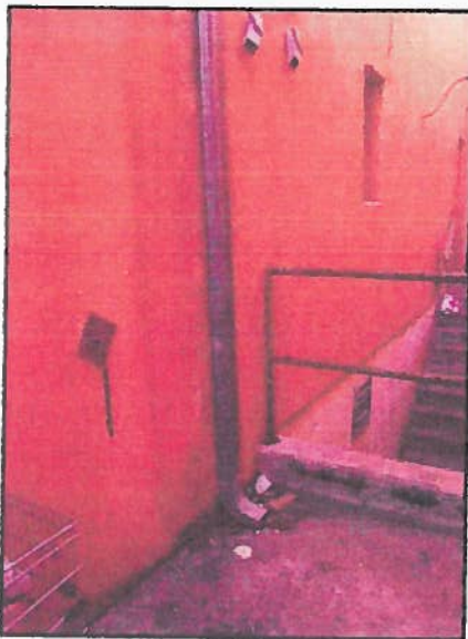
Fig. 4. Gutter spilling into alleyway.
