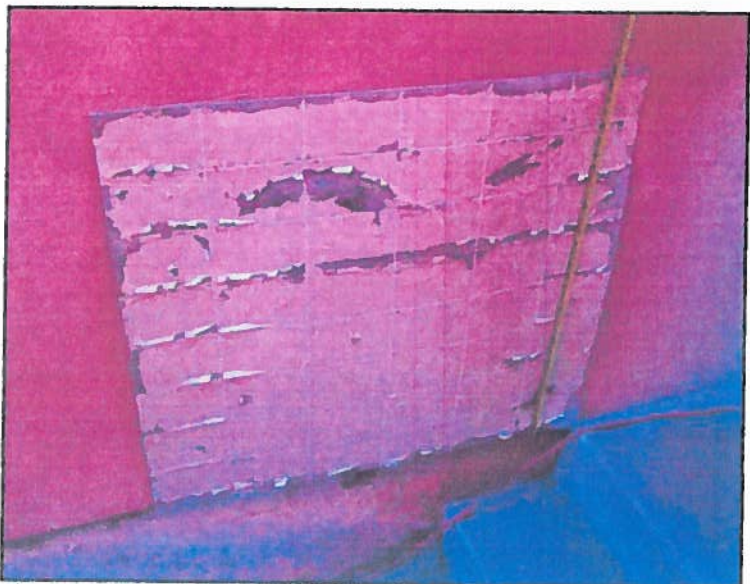
Fig. 30. Coated masonite sheet covering plumbing repair on exterior plaster wall.
