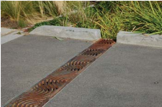
Decorative Grill and Curb Cut
