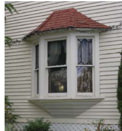
Oriel: Project from the side of a building, like a bay window, but are supported by brackets.
