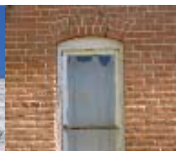
Segmented brick arch over double-hung window
