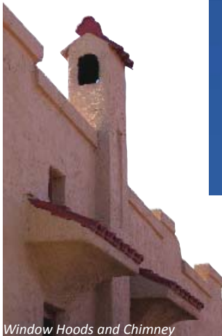
Window Hoods and Chimney
