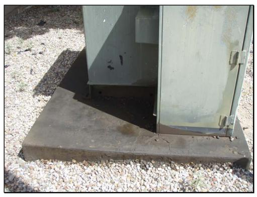
No. 21 – View of staining at the concrete base of the pad-mounted transformer located at the southern property boundary of the North Area.
