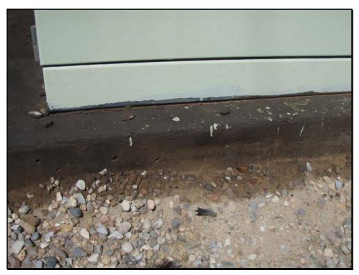
No. 22 – View of staining at the concrete base of the pad-mounted transformer and surrounding surficial soils located at the southern property boundary of the North Area.
