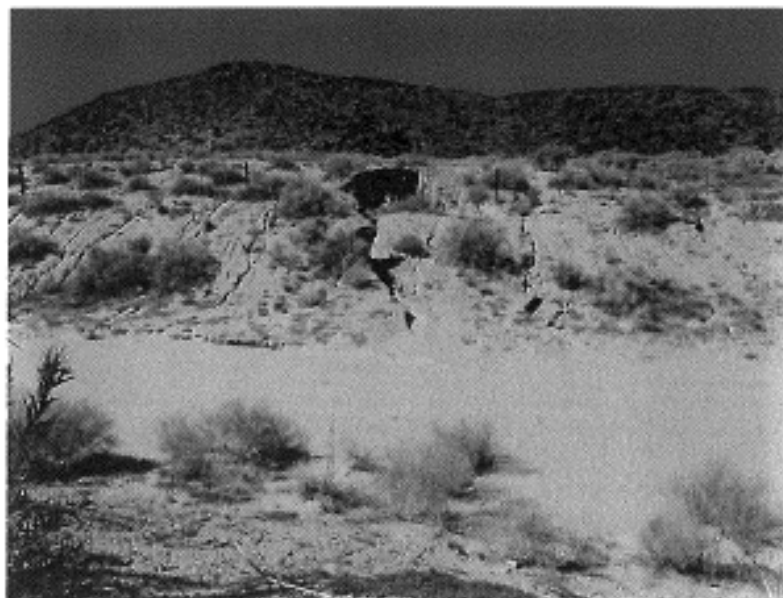
Figure 8: Example of second failed detention pond between roadway and Petroglyph National Monument fence ((further west on Lava Bluff Drive, Taylor Ranch)
