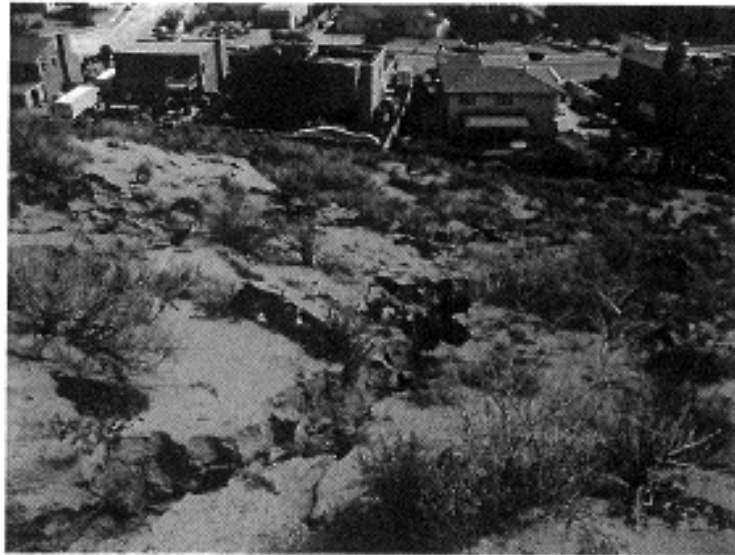
Figure 3. Example of failed rear yard walls at base of escarpment (Painted Pony Drive, Taylor Ranch)
