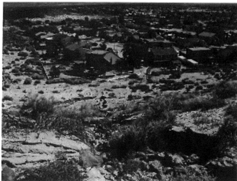
Figure 4: Example of failed rear yard walls at base of escarpment (Painted Pony Drive, Taylor Ranch)
