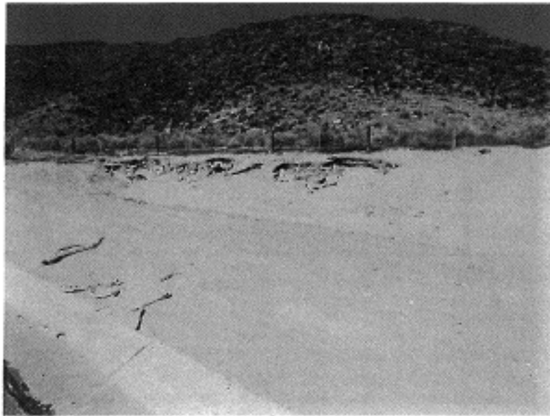
Figure 7: Example of failed detention pond between roadway and Petroglyph National Monument fence ((Lava Bluff Drive east of Unser, Taylor Ranch)
