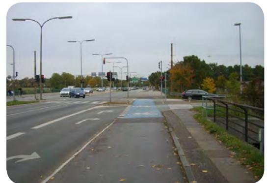
At this unsignaled right turn, the cycle track has dropped to a bike lane with blue coloration and pavement markings through the conflict area.
