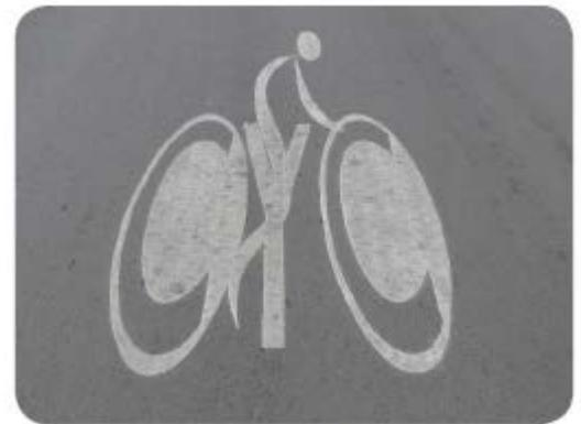
Figure 9 - Bicycle Boulevard pavement marking.
