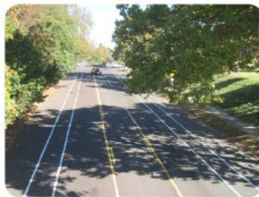
This road was re-striped to convert four vehicle travel lanes into three travel lanes with bike lanes.
