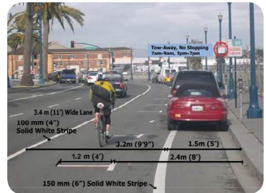
Floating bike lane when parking is allowed on The Embaradero, San Francisco. Source: sfmta.org
