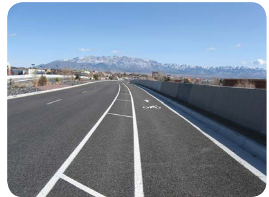
Buffered bike lanes protect cyclists from fast-moving traffic.
