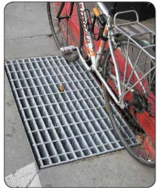
Examples of bicycle-safe drainage grates.
