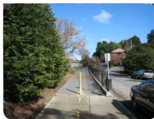
Bollards and pavement change prevent motor vehicles from using the trail.
