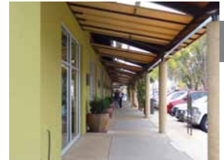
Portal on the West Side
