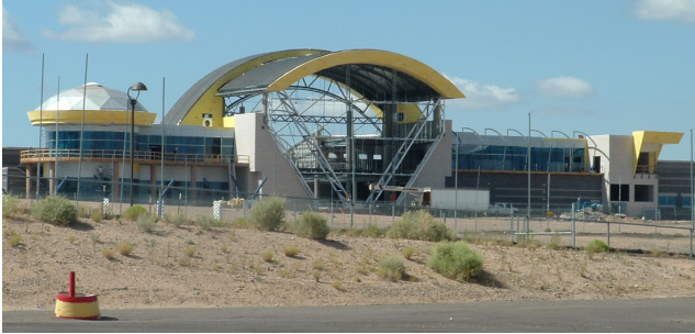
Balloon Museum under construction
