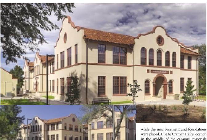
This \$6.4 million project consists of a remodel of the historic 1928 classroom building and an addition of a new classroom building wing. The construction team made structural modifications, updated HVAC and plumbing, added fire protection and contemporary communications such as computer connects and video conferencing.
