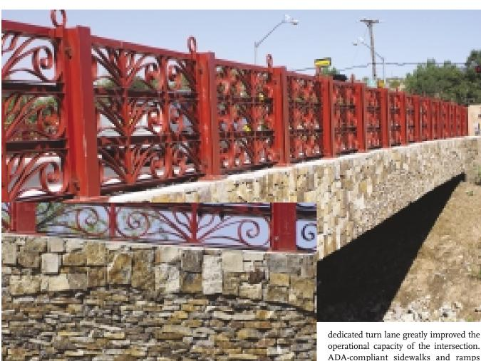
**Situated in the heart** of one of Santa Fe's oldest neighborhoods, Camino Alire provides one of few connections to the rest of the city. The original Camino Alire Bridge, constructed in 1958 over the Santa Fe River, was a 3-span channel beam bridge supported by piers on foundation piles. The new bridge, completed in April 2007, is a single-span, pre-stressed concrete, box beam bridge. This construction
