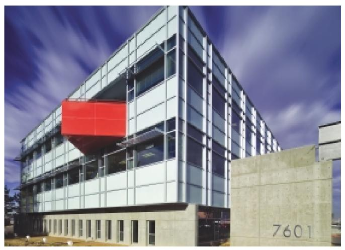
At three stories and 85,000 sq ft, New Mexico's first LEED gold commercial building focused on incorporating meaningful sustainable features in order to use 30% less water and 45% less energy than a typical structure. High-performance glazing is shaded by integral external horizontal shades to balance daylight penetration with energy efficiency. A direct-indirect evaporative cooling system provides efficient operation and an option for "free" cooling using outside air. With an under-
