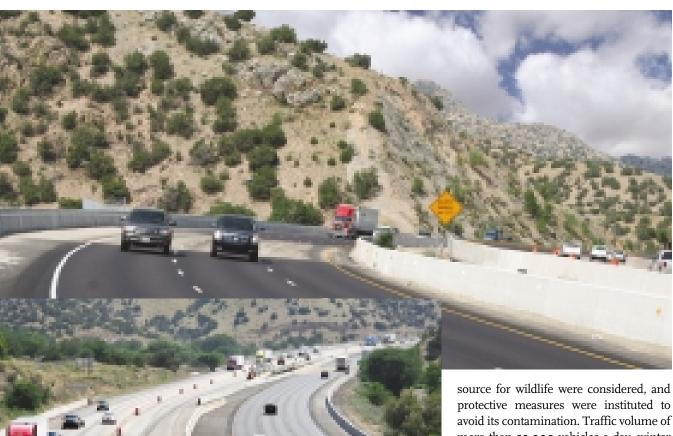
This transportation corridor bisects the Rocky Mountain range, an area that provides for wildlife habitats. Vehicle-wildlife collisions were a concern in the area, so the 4.2-mi project was undertaken to rehabilitate seven bridges, improve drainage and signage, construct barrier walls, median breaks, and wider shoulders, and create, for the first time in the state's history, special fencing to protect wildlife.
