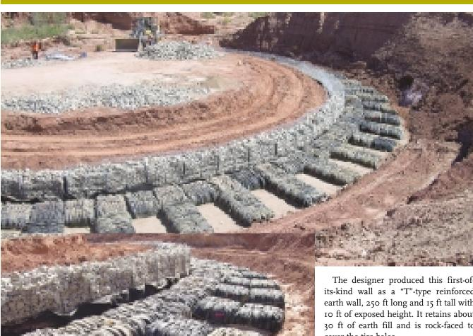
The construction team on this project found a unique solution to erosion control: roll out used tires to stop an arroyo from eroding a right of way.
