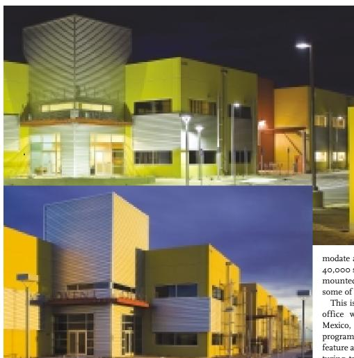
The developer of the 12,900-acre Mesa Del Sol employment center in southeast Albuquerque wanted a high-tech sustainable design for its first building: the 87,600-sq-ft Advent Solar warehouse. The resulting \$4.9 million shell is designed to draw equally-minded tenants to the center. A galvanized, corrugated metal tower at the northeast corner promotes industrial high-tech aesthetic while serving as the entryway.
