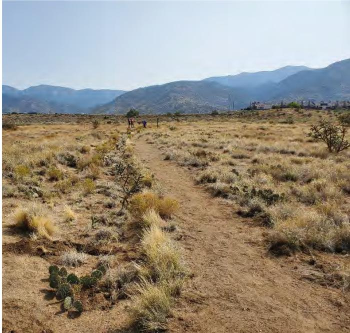
*Recently constructed by a Boy Scout group, this is an example of “bumping up” an eroded trail to take advantage of higher ground and improved runoff. The closed trail is just to the left of the new trail.*
