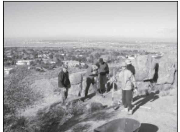
FHVHA volunteers digging holes through granite
