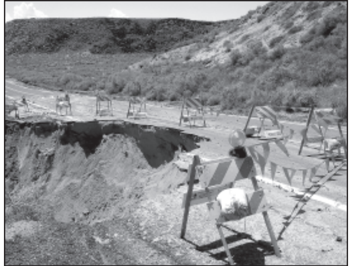
Road damage from summer rains in Boca Negra Canyon
