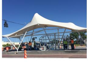
The canopy at Central and Coors is the first one to be installed along the ART route. FabriTec Structures of Dallas, Texas is handling the canopy installations, utilizing marine-grade steel for the framework. The caniopies themselves are made of polytetrafluoethylene, a Teflon®-coated, woven fiberglass membrane that is extremely durable and weather resistant. The canopies are designed to stand up to scorching desert heat, and are fire-resistant, as well.
