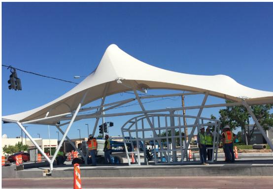
The canopy at Central and Coors is the first one to be installed along the ART route. FabriTec Structures of Dallas, Texas is handling the canopy installations, utilizing marine-grade steel for the framework. The canopies themselves are made of polytetrafluoroethylene, a Teflon®-coated, woven fiberglass membrane that is extremely durable and weather resistant. The canopies are designed to stand up to scorching desert heat, and are fire-resistant, as well.
