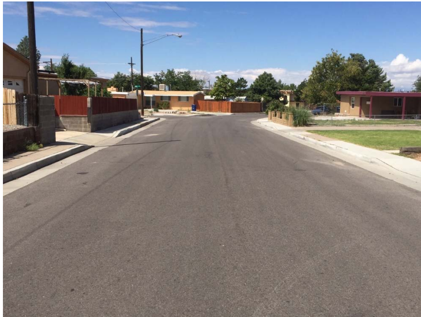
Figure IV.B.3 Baldwin Avenue west of Elizabeth Street
