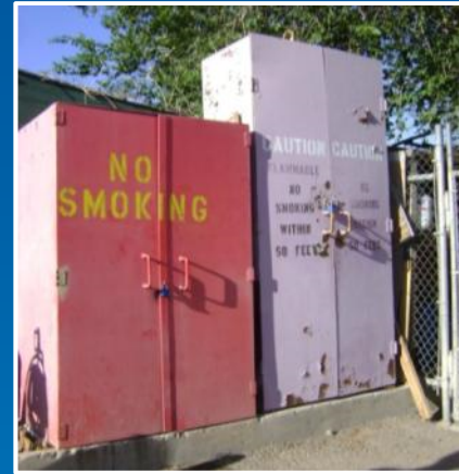
Flammable materials should be stored in well labeled flammables cabinets.
