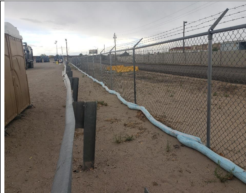
Stormwater Control Measures – Wattles on East Perimeter of Blue Fleet Lot.
