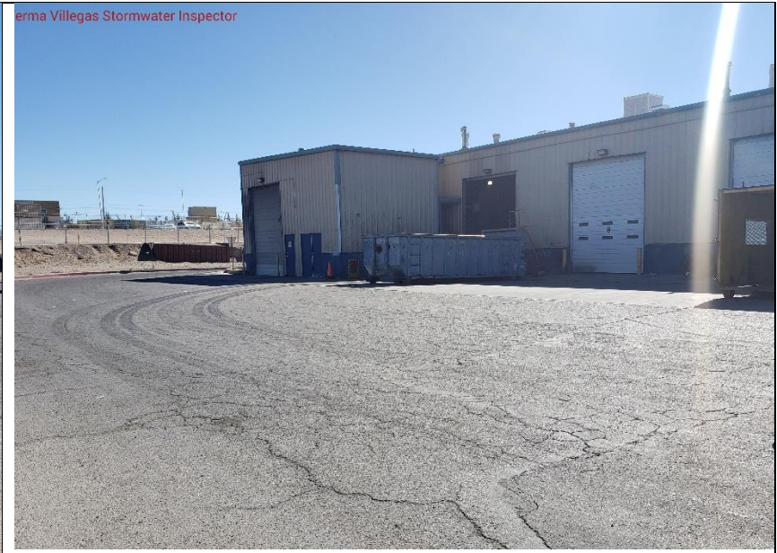
Wash Building and Tire Storage
