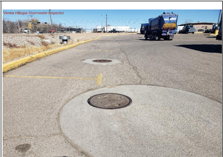
Stromceptors and Detention Pond West of Blue Fleet Parking
