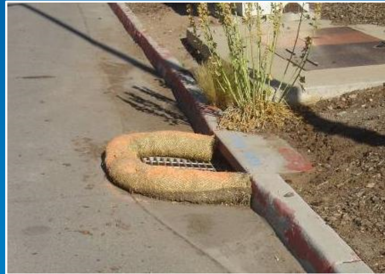
Straw roll installed to protect a storm drain.
