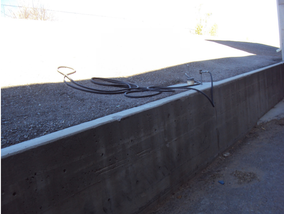
IMG_367: Hose bib and hose for trailer spray down
