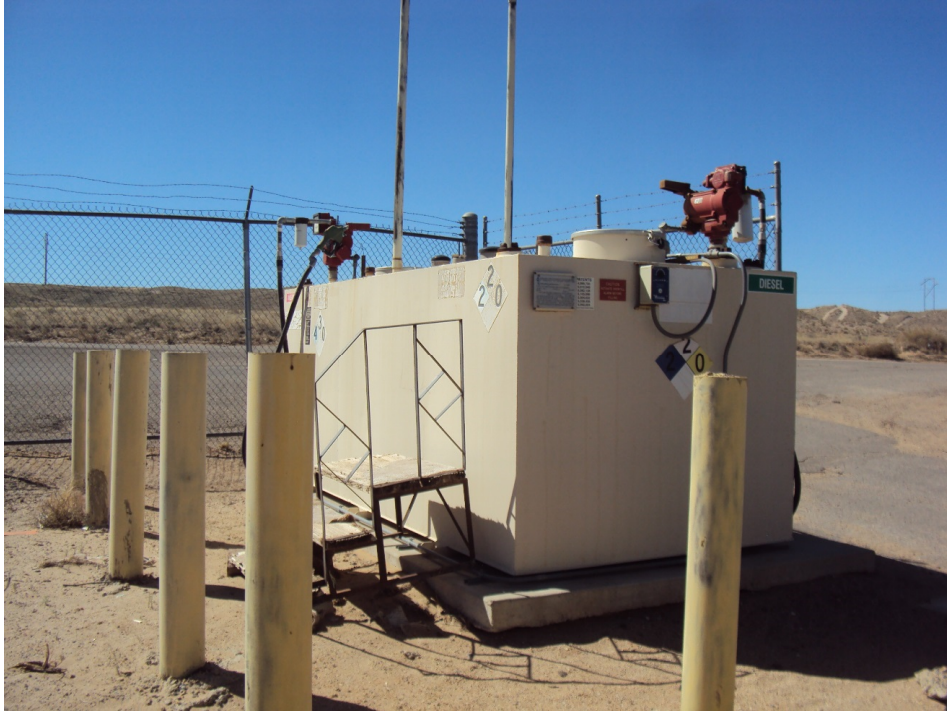
IMG_385: Fuel storage tanks (Unleaded not in use)
