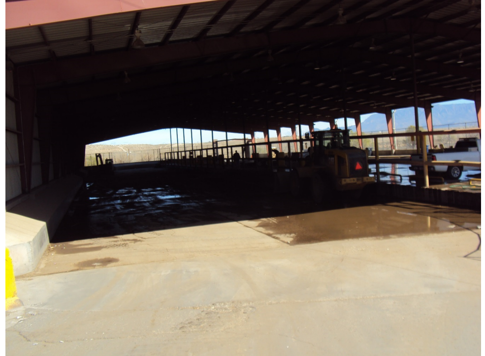
IMG_368: Tipping floor
