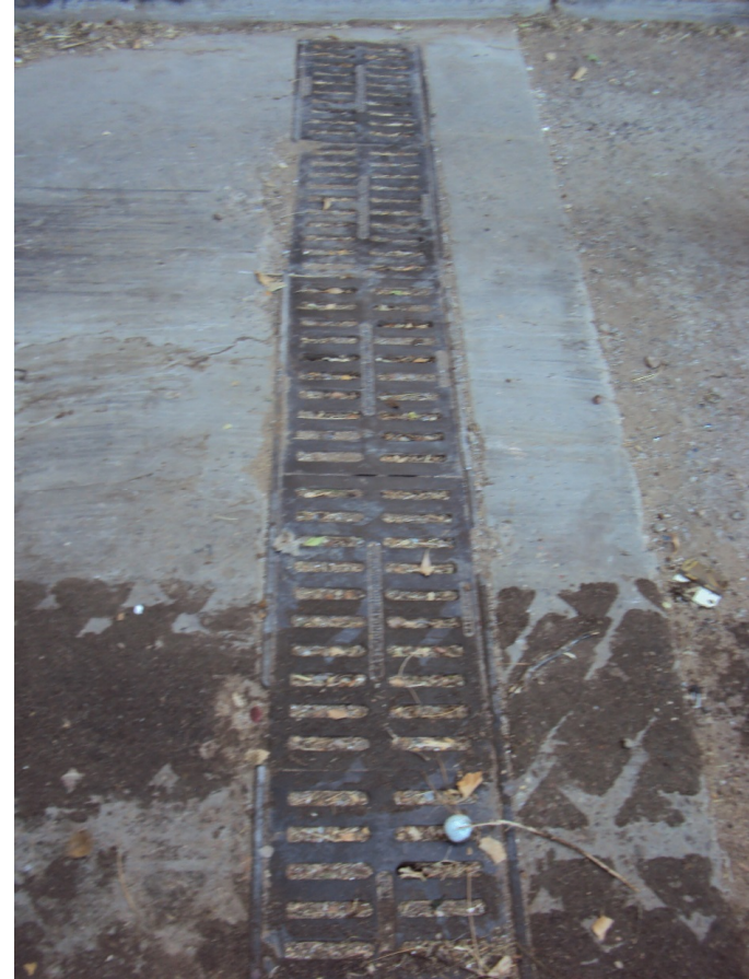
IMG_366: Trench Drain under the truck loading area
