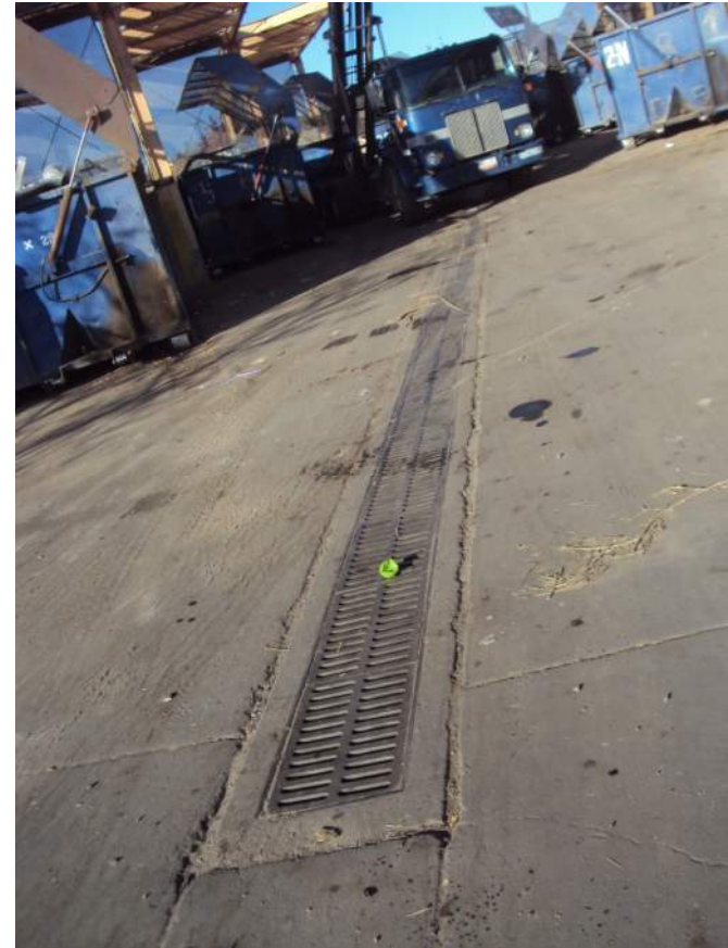
IMG_142: Trench drain
