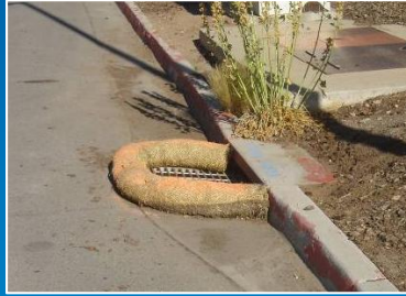
Straw roll installed to protect a storm drain.
