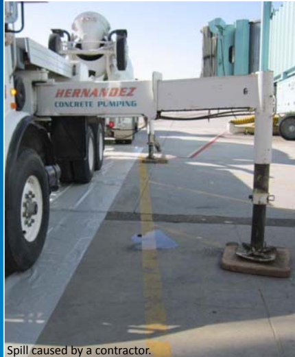
Spill caused by a contractor.
