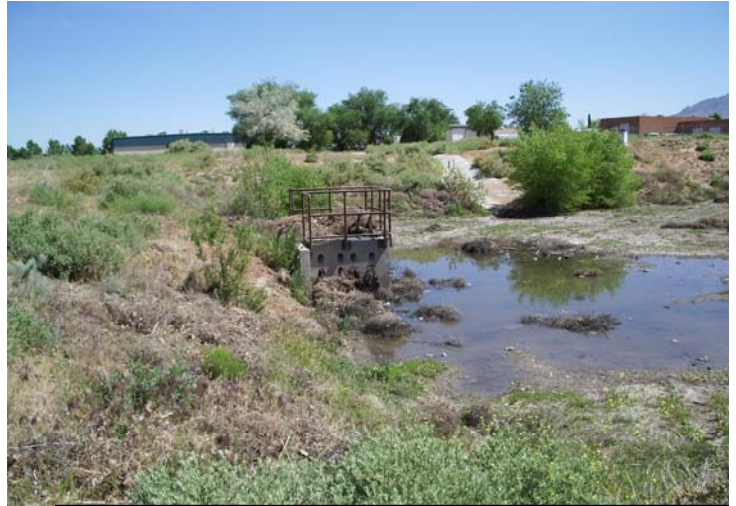
Pino Arroyo Debris Basin reverse slope ported outlet.
