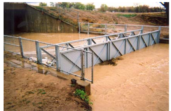
La Orilla Debris Baffle (4/3/04)
