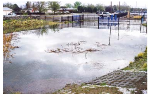
Haynes Park Debris Forebay (Bank full - 4/3/04)
