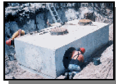
Nutrient Separating Baffle Box
