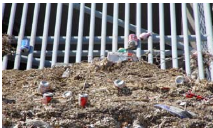
Trash Rack Detail – South Broadway Pond (4/23/04)
