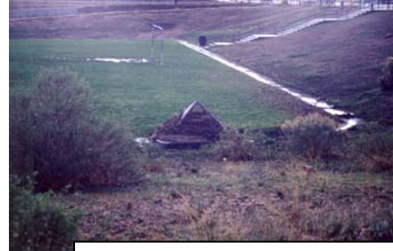
Highland Detention Basin Trash Rack (4/3/04)
