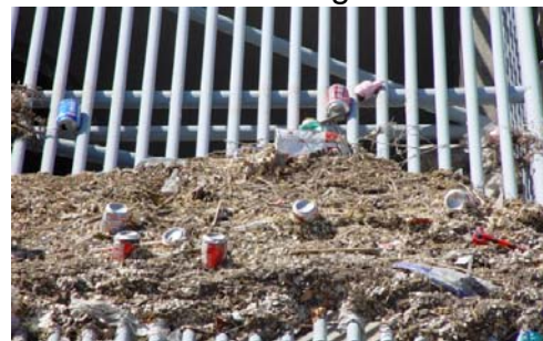
Trash Rack Detail – South Broadway Pond (4/23/04)
