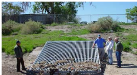
Trash Rack – South Broadway Pond (4/23/04)
