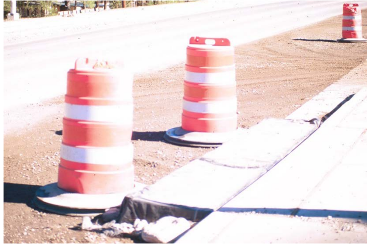
Curb drop inlet protection in urban area – Type II
