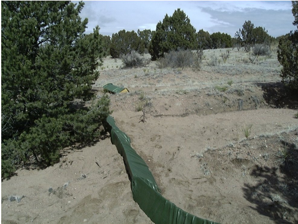
Triangular sediment filter dike
