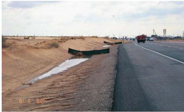
Check dams at roadside ditch
