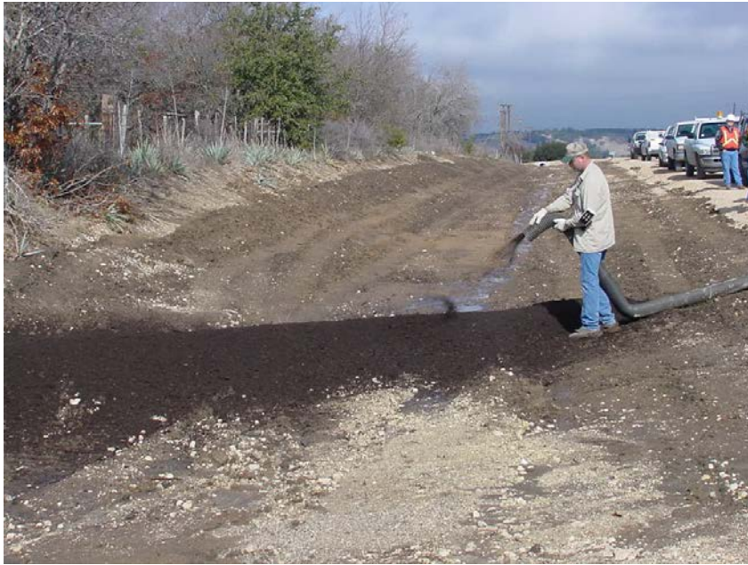
Compost berm under construction
