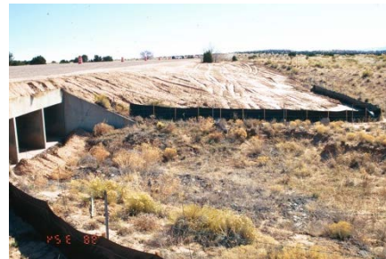
Silt fence at outlet of box
