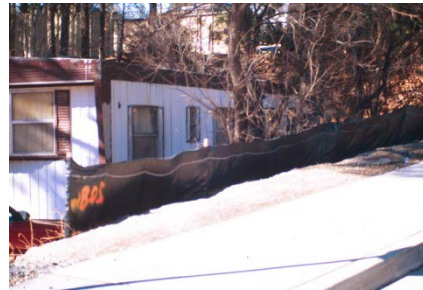
Silt fence in urban area
