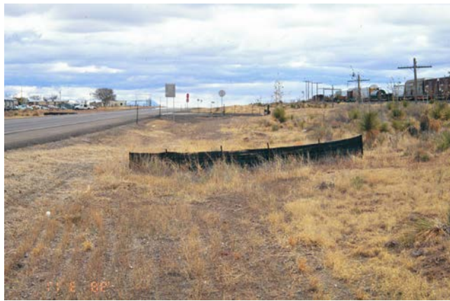
Check dam at roadside ditch
