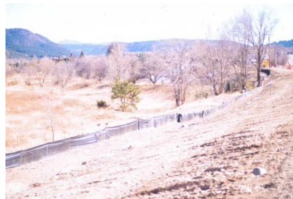
Silt fence in rural area
