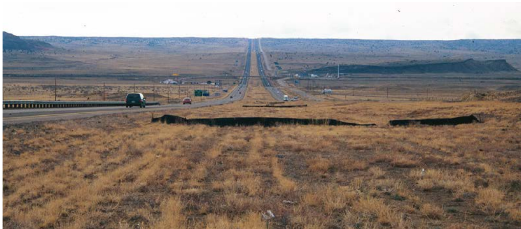
Check dams at median
