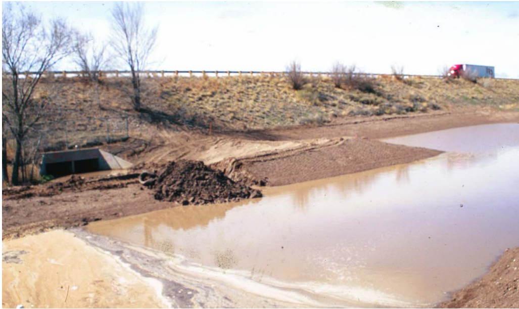
Sediment pond at inlet of box
