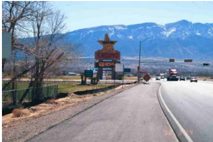
Silt fence in urban area
