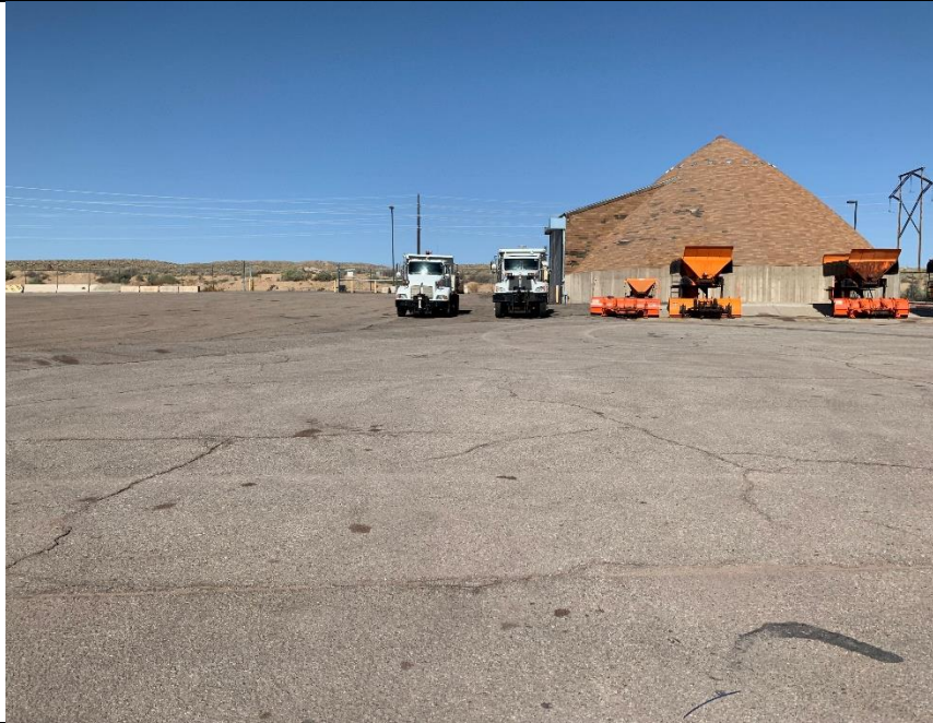
Salt Storage Building
