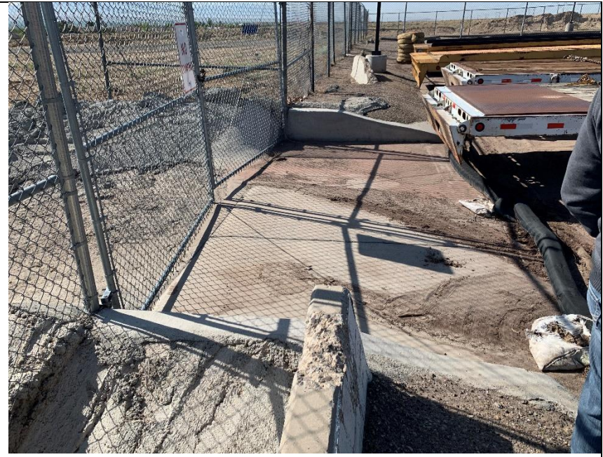
Location where storm water discharge leaves site.
