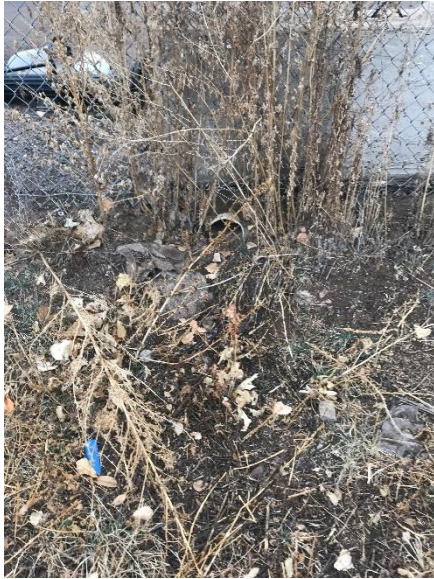
No Flow at Outfall BP1
