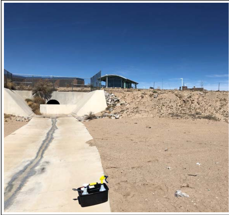
5. Pond 1A sample location, view toward the northwest
