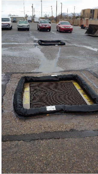
Flow at Outfall SS1A
