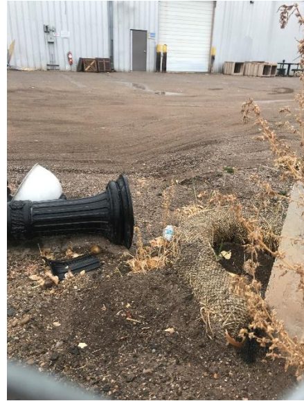
Wattle at Outfall BP1
