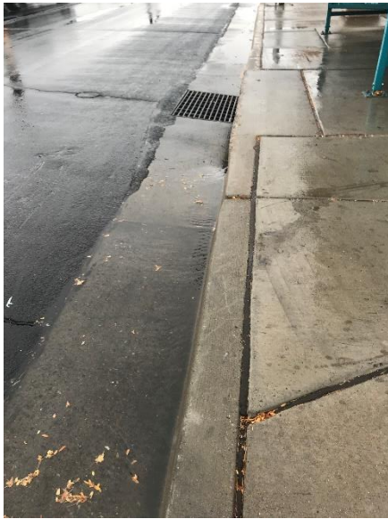
Flow at Outfall FS1
