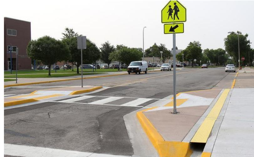
Figure 25: Raised Crosswalk with Curb Extension and In-Street Pedestrian Crossing Sign
