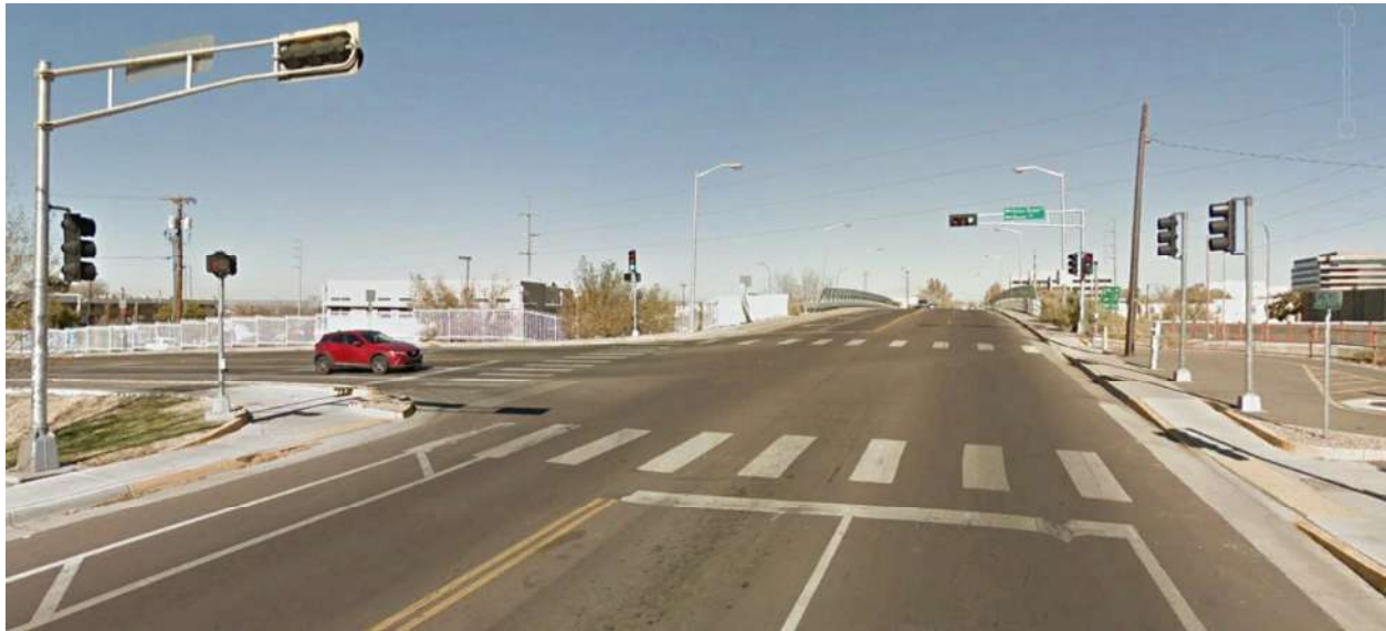
Photo 8- Signalized T-Intersection at San Pedro Dr / Haines Ave
