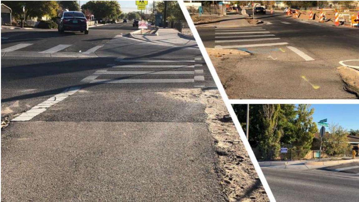
Photo 2- Existing Non-ADA Compliant Curb Ramps
