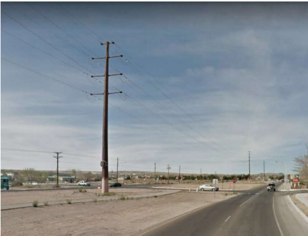
Photo 3- Existing Transmission Poles in Median
