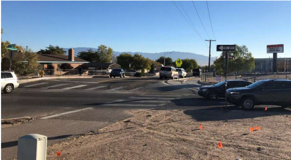
Photo 4- Crosswalk Striping and School Zone Beyond Intersection
