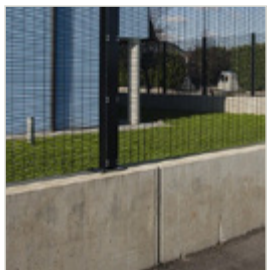
Welded wire fabric fence with board form concrete base
