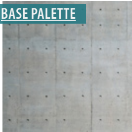
Board form concrete base
