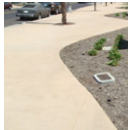
Warm colored concrete
