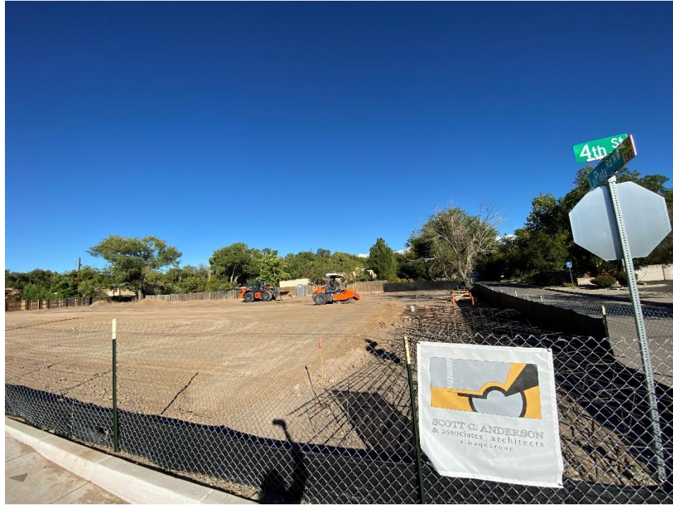
View from W Property Line, looking NE towards adjacent neighborhood
