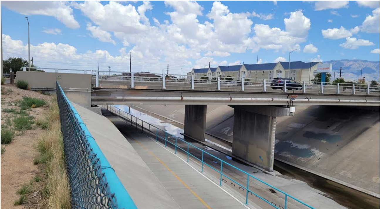
North Diversion Channel Multi-Use Trail.
