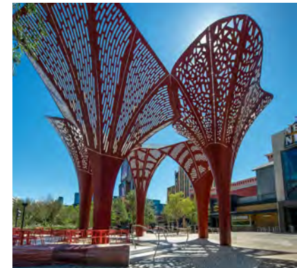
Shade Structure and Seating in Las Vegas, NV
