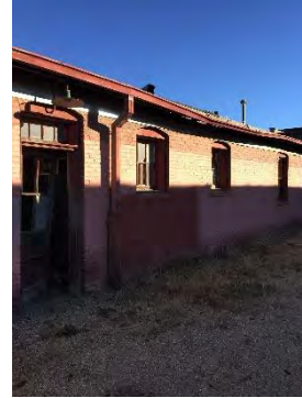
Figure 2 Exterior of North Wash Room
