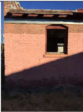
Figure 3 Window Exterior of North Wash Room
