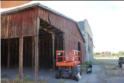
Figure 3, Sheet Metal House, NE Corner
