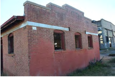
Figure 1 Front Exterior of North Wash Room
