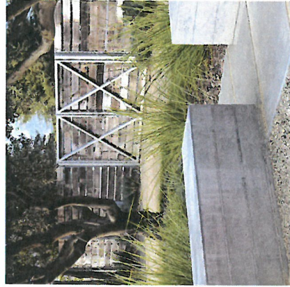
BOARD FORM CONCRETE VERTICAL WALLS
