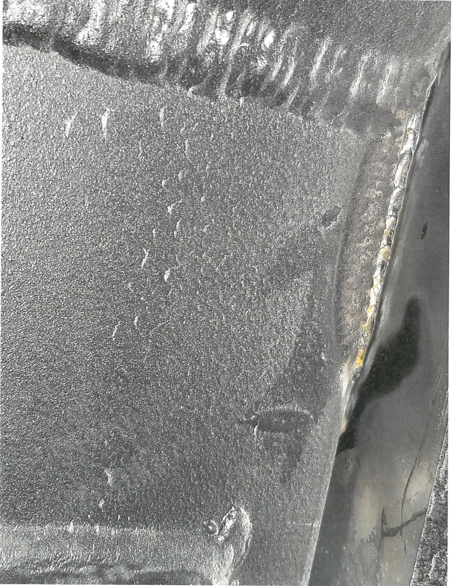
1708 - Rear Frame cross plate rusting and welds are not bonded
