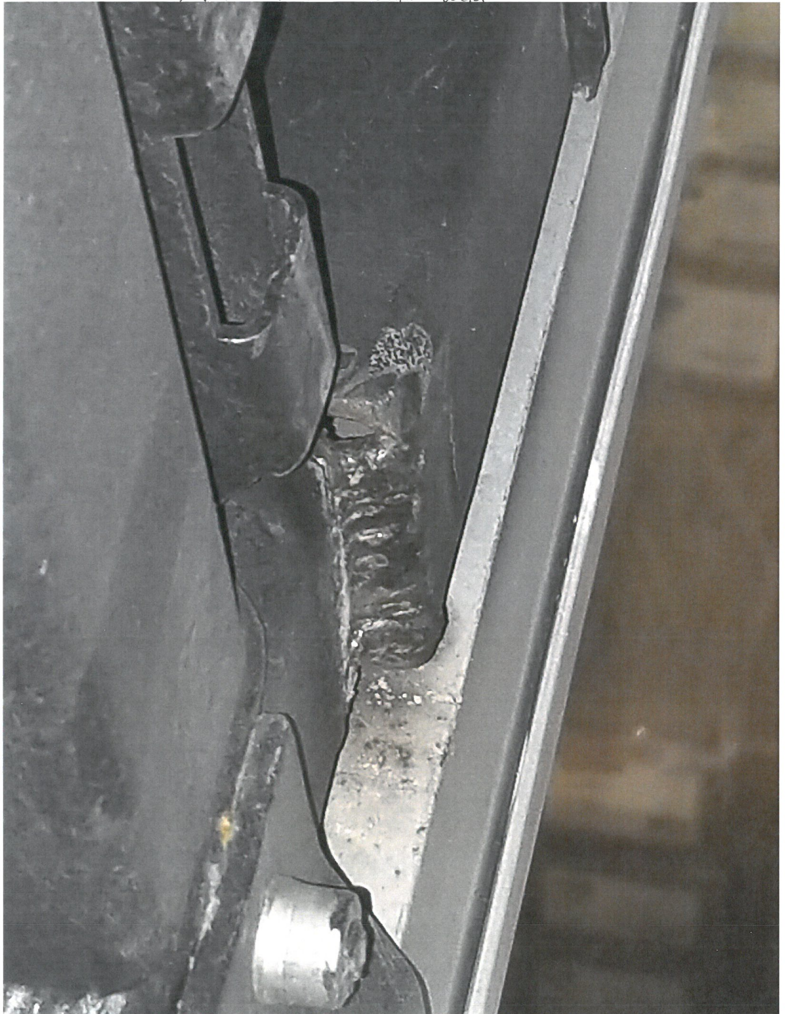
1706 C/S Bridge plate Center door incomplete weld
