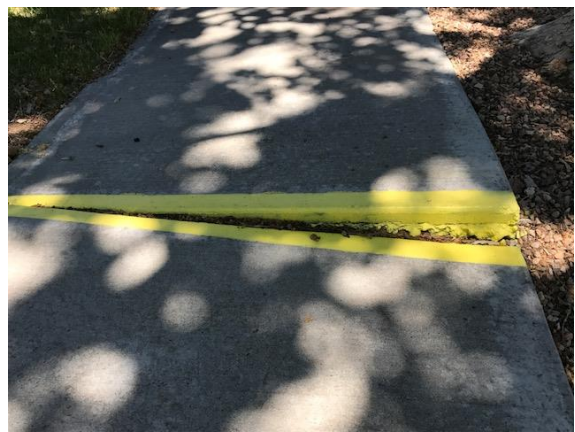
This image depicts an uneven surface of a sidewalk that has been painted – this appears to be done in lieu of actually replacing this section of sidewalk, but it does not correct the violation and remains a hazard to a person in a wheel chair or without vision. (Address: 8500 block of Canyon Run Rd NE, COA)
