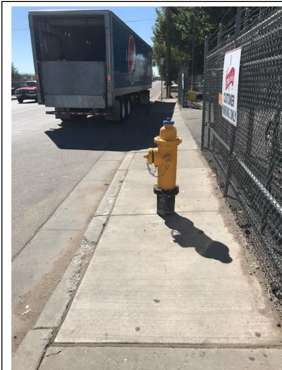
This image depicts a fire hydrant obstructing the sidewalk, which creates a hazard for people in wheelchairs or individuals with vision impairments. Note: This obstruction is near the utility pole depicted in the other image. (Address: 1700 block of 2nd Street SW, COA)
