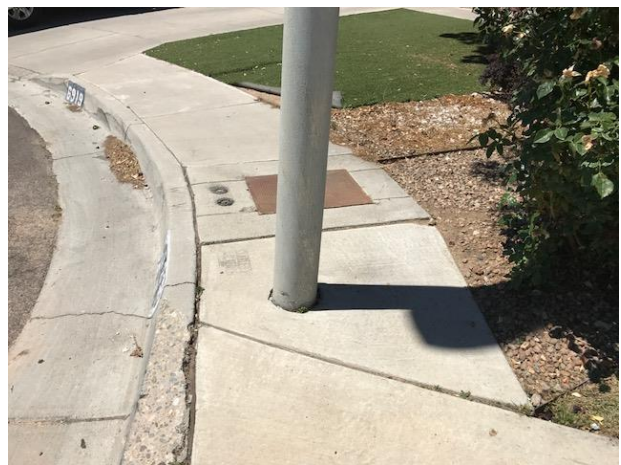
The photograph on the left depicts a sidewalk with a light pole blocking the pathway – a wheelchair would not be able to pass through. (Address: 6900 block of La Lucena Ave NE, ABQ)
