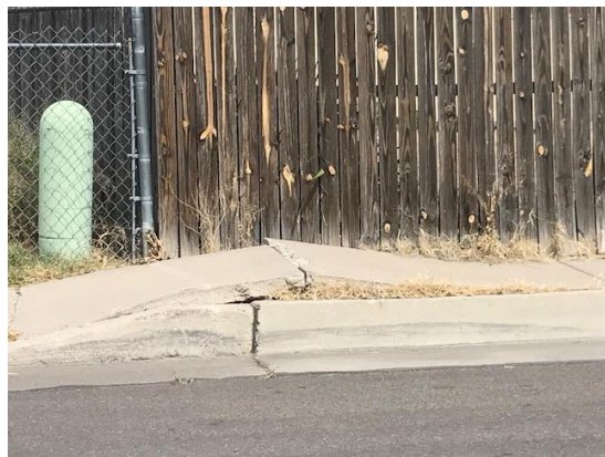
This image depicts an example of a common problem with many sidewalks in the City. This buckled sidewalk is especially concerning, because the two segments do not evenly come together, but instead present a more difficult situation for a wheel chair bound person or a person with vision impairment. (Address: 900 block of Field St SW, COA)
