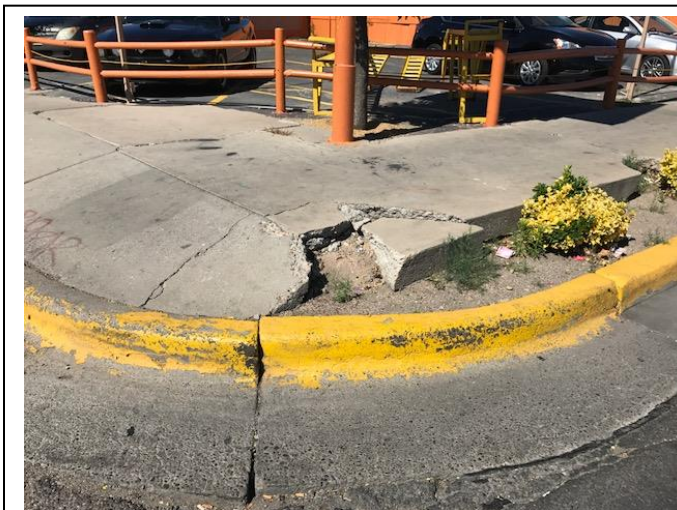
This photo depicts a situation that has two blatant violations. The curb does not have an ADA ramp and the sidewalk is severely damaged. This situation is unsafe to both disabled and able bodied individuals, especially elderly citizens. Unfortunately, this photo doesn't sufficiently capture the steep angle of the sidewalk that adjoins the curb, which creates even further risks. (Address: 7500 block of Central Ave NE, ABQ)
