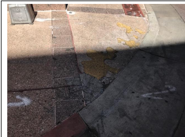
This image depicts a corner in downtown where the tactile surface has been worn down and is in need of replacement.
