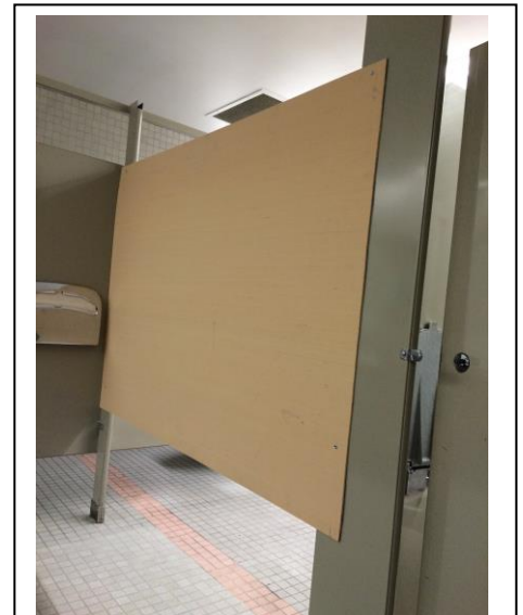
This was an attempt to widen a non-compliant women's bathroom on the basement level of City Hall, but is still missing ADA required grab bars and is unprofessional in appearance.
