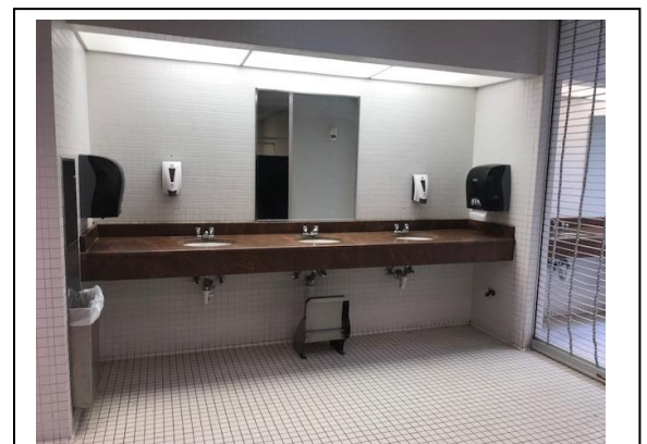
This is an example of a non-compliant bathroom at the COA BioPark Zoo. Sinks for disabled persons in wheel chairs should not be mounted higher than 34 inches from the floor, and allow a 29 inch clearance.
