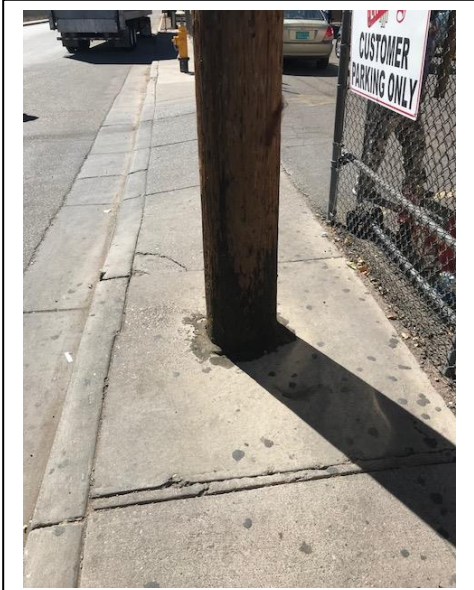
This image depicts a utility pole obstructing the sidewalk, which creates a hazard for people in wheel chairs or individuals with vision impairments. (Address: 1700 block of 2 nd Street SW, COA)
