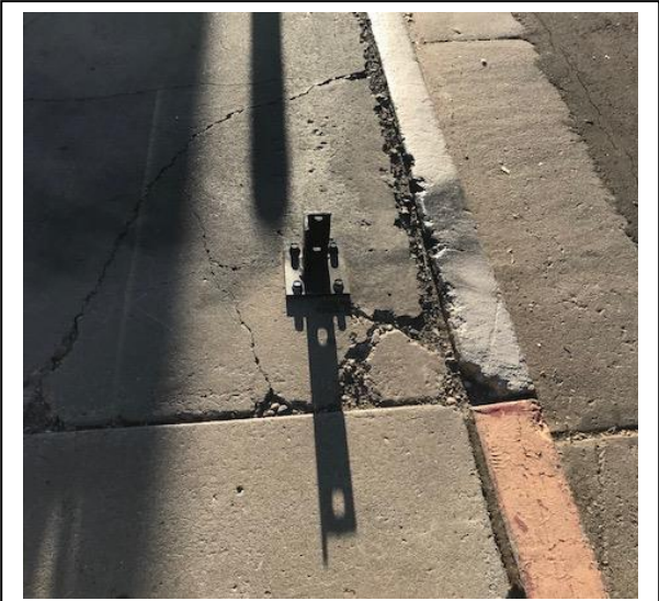
This is an example of a potentially dangerous obstruction on the sidewalk on Tijeras Avenue NW, just south of the old County building, adjacent to the Civic Plaza. This obstruction poses a hazard to both sighted and non-sighted individuals.
