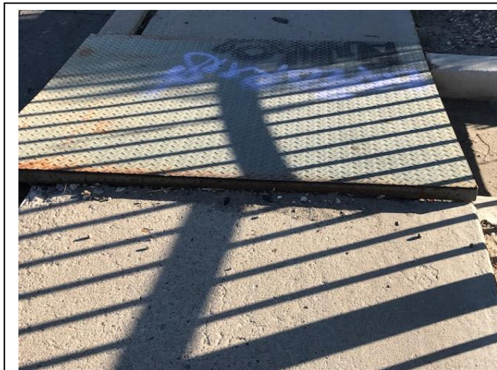
This image depicts a metal plate laid over a drainage ditch, but causes an uneven surface for individuals with visual impairments and in wheel chairs. (Near the intersection of Broadway Ave NE and Kinley Ave NE, COA)
