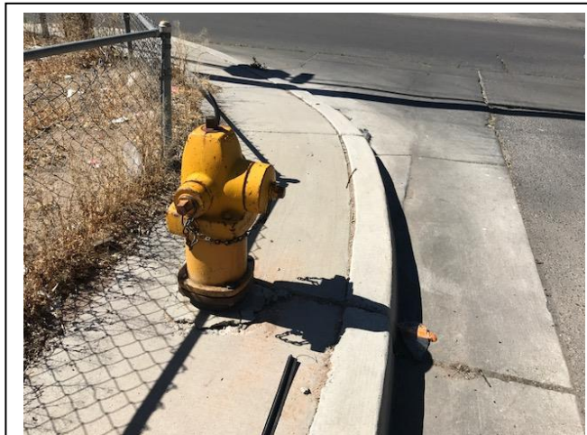
This image depicts a fire hydrant that blocks the path and thereby obstructing the way for a wheelchair bound person or a blind person to safely navigate. (Address: 100 block of Mesilla St NE, COA)
