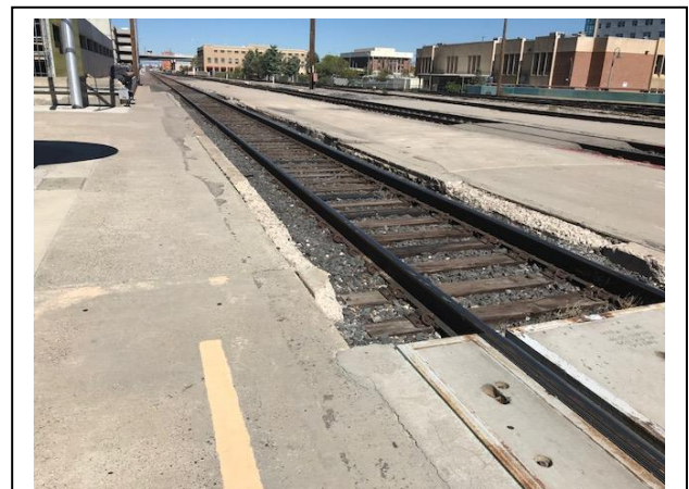
This pedestrian area at the COA Transit Center does not have any detectable warning signs for blind individuals, to ensure they do not unknowingly walk over the tracks or off the platform edge.
