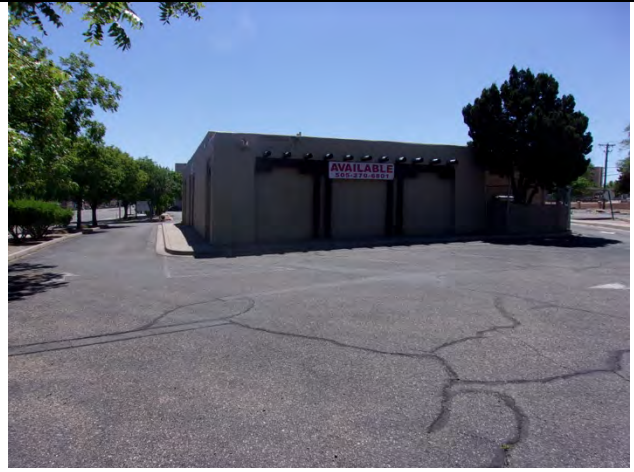
Photo 2: View southeast across the subject property.
