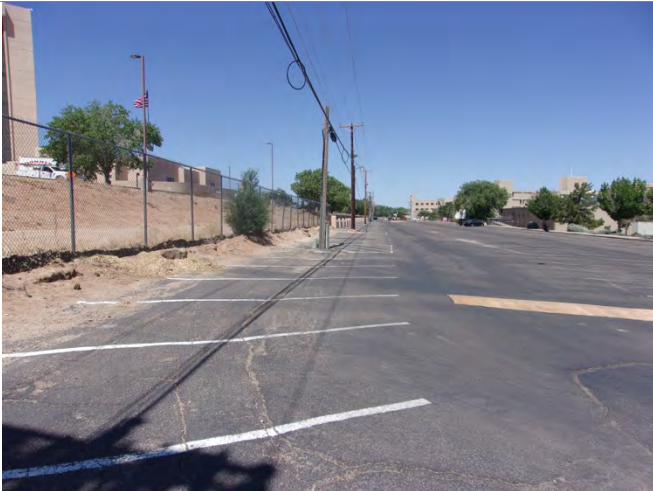
Photo 5: View northwest along the south side of the subject property.
