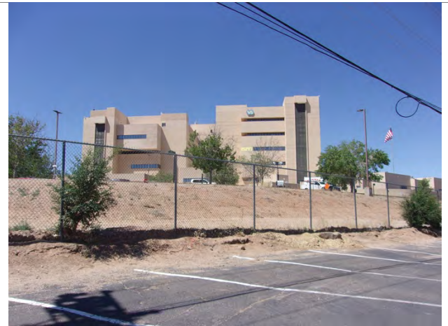
Photo 22: View off-site south towards the VA Hospital.
