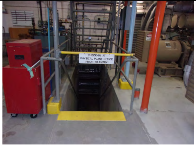
Photo 14: Basement (confined space) inside the powerplant.
