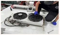
AFR Technician Jason Zamora replacing condenser fans to ensure our crews have a working HVAC system for the hot summer months.
