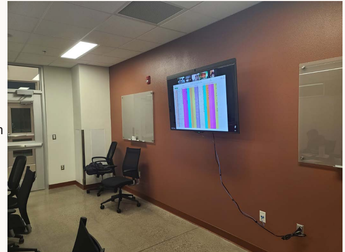
New DTEN interactive monitor at Fire Station 9.
