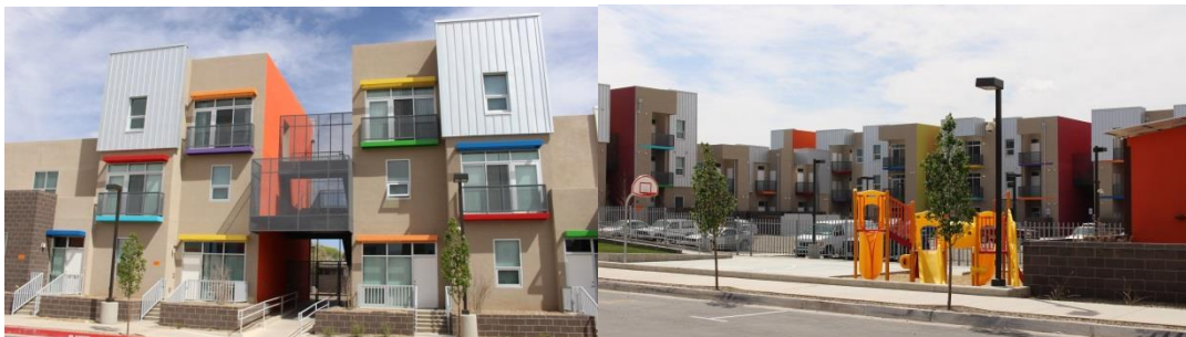
PLAZA CIUDANA- Located at 312 Indian School Rd NE, Albuquerque, NM 87102, the project consisted of the construction and management of a one, two, and three-story
