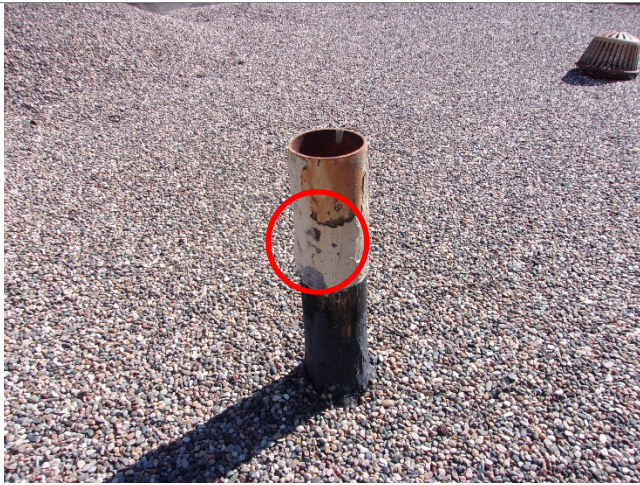
Photo 9: Sample No. 48-A8 of roofing vent penetration tar contained 3% chrysotile asbestos.
