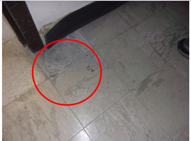
Photo 10: Sample No. 48-A12 of 9"x9" floor tile with black mastic in the basement contained 2% and 4% chrysotile asbestos, respectively.
