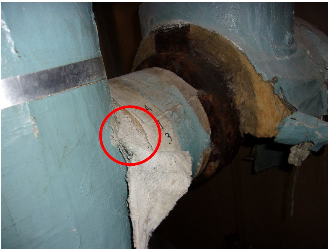
Photo 11: Sample No. 48-A13 of "hard" white powder TSI elbow contained 3% chrysotile asbestos.
