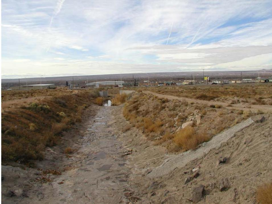
*No. 49 – Looking west and down the drainage channel from the Kirtland Addition subdivision. Note rebar and concrete in sidewall of drainage on the right side (north) of the picture.*
